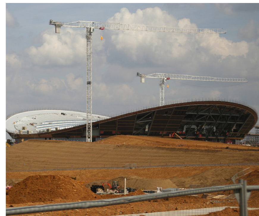
Construction of the 2012 Olympic Velodrome
