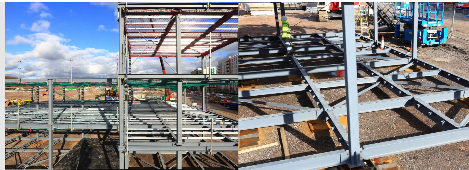
This entirely deconstructable steel frame by ES Global forms a temporary marketing suit, Chobham Manor in London. The majority of the structure could be re-used elsewhere providing significant environmental savings, this combined with faster construction times provides clear benefits that could be extended beyond the temporary structures market.
