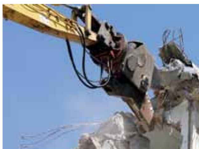
A delicate tool for smashing the façades off buildings
