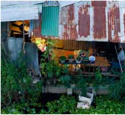
Inventive reuse of steel
