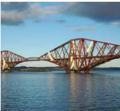
The well-painted Forth Road bridge
