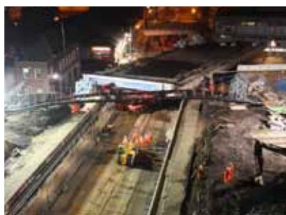
Caversham Road Bridge 13
