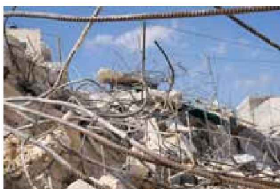
Reinforcing steel in a demolished building
